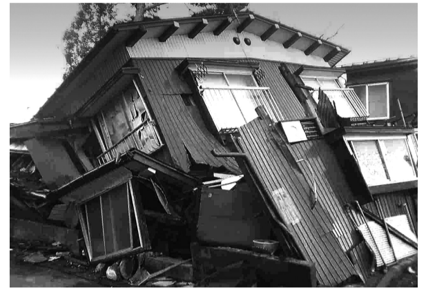
House destroyed in the Niigata-Chuetsu Earthquake (July 2007, Ojiya City)
